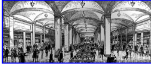
The East Traction Concourse Room.
